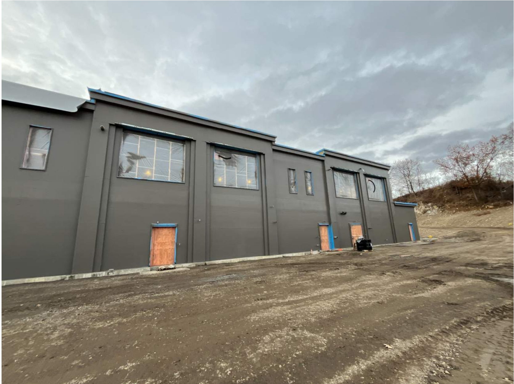
Building Envelope at Service Area 12/19/24
