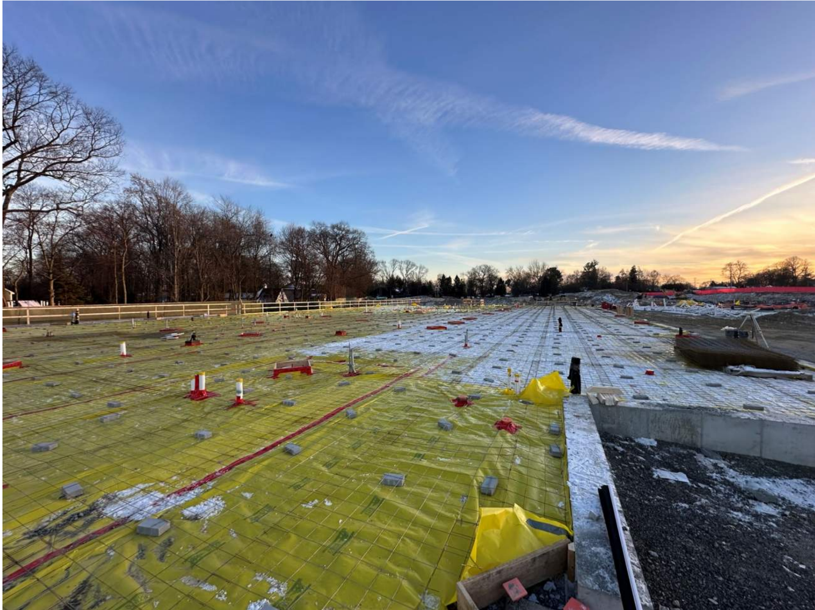
Slab on Grade Prep 12/23/24
