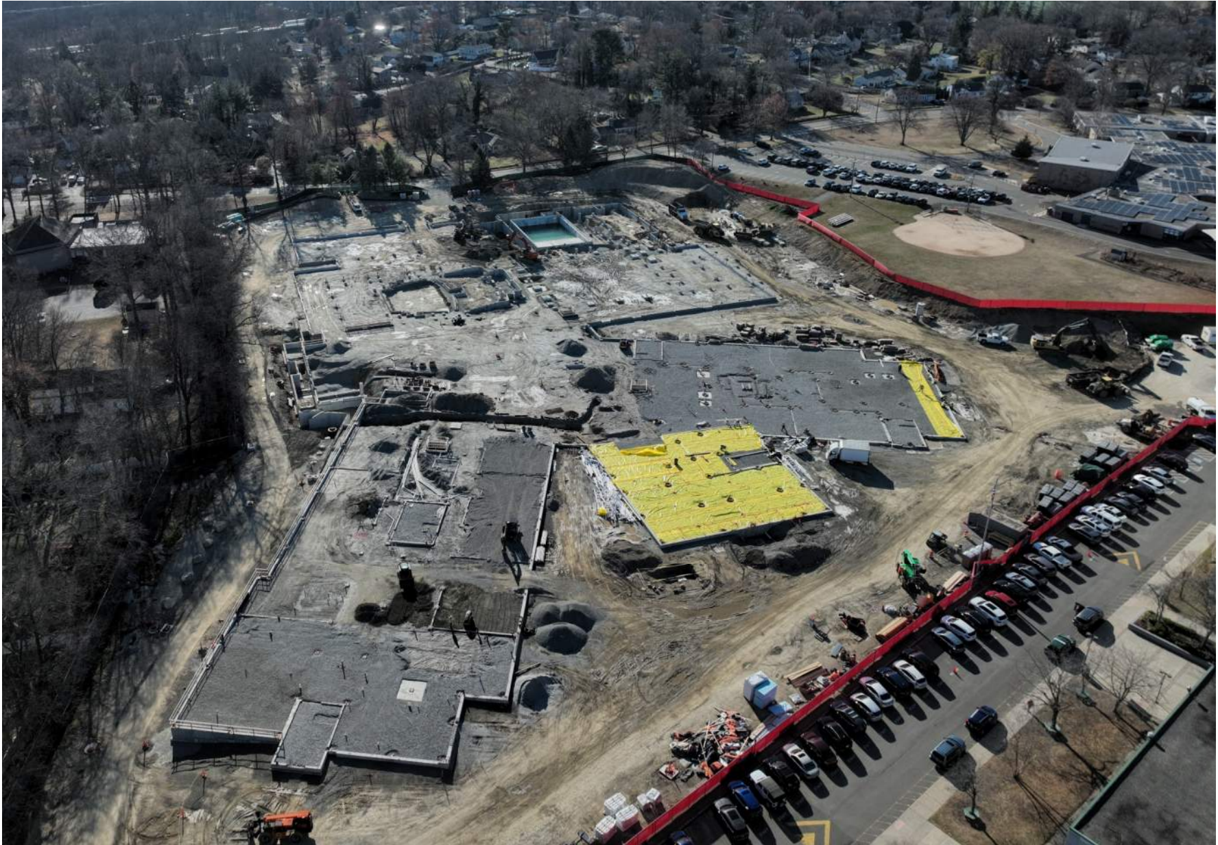
Drone Image – Foundations, Underslab Utilities, Pool Concrete 10/31/24
