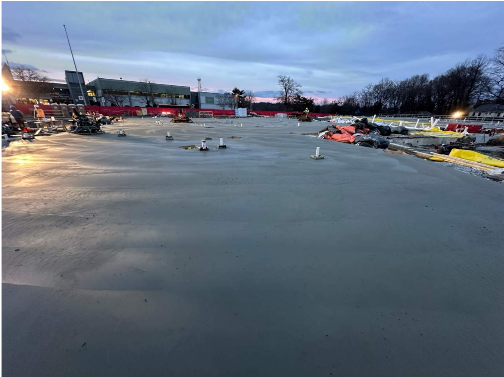
Concrete Slab on Grade 12/19/24
