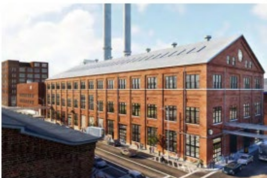
Figure 37. Brooklyn Navy Yard Building 127 (Brooklyn, NY)
