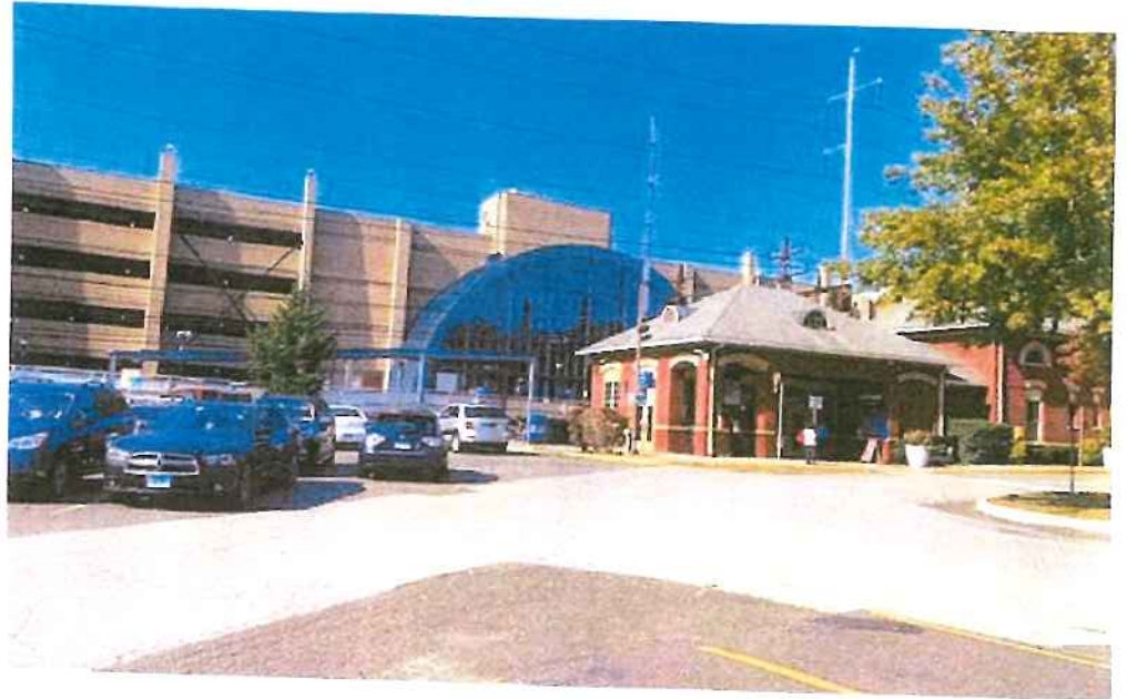
Adjacent Train Station Building & Parking Garage
