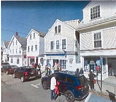
Figure 3C: Rockport, MA. Source: Google Street View
