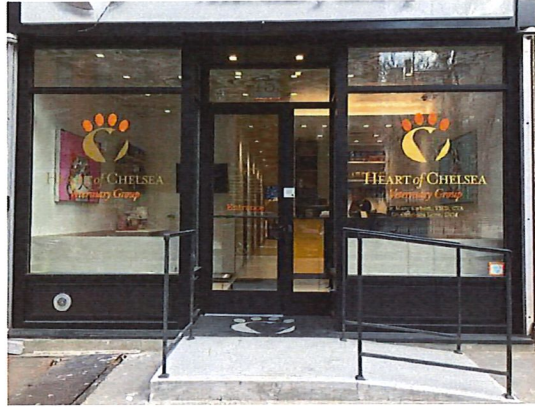
Figure 12: Contemporary Storefront Source: Skywindowsnj.com
