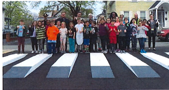
Figure 23: 3-D Painted Crosswalk Source: Mayor's Office, City of Medford, MA
