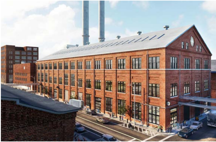
Figure 37. Brooklyn Navy Yard Building 127 (Brooklyn, NY)
