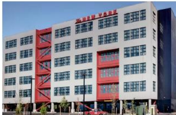
Figure 38. New York Building (Portland, OR)
