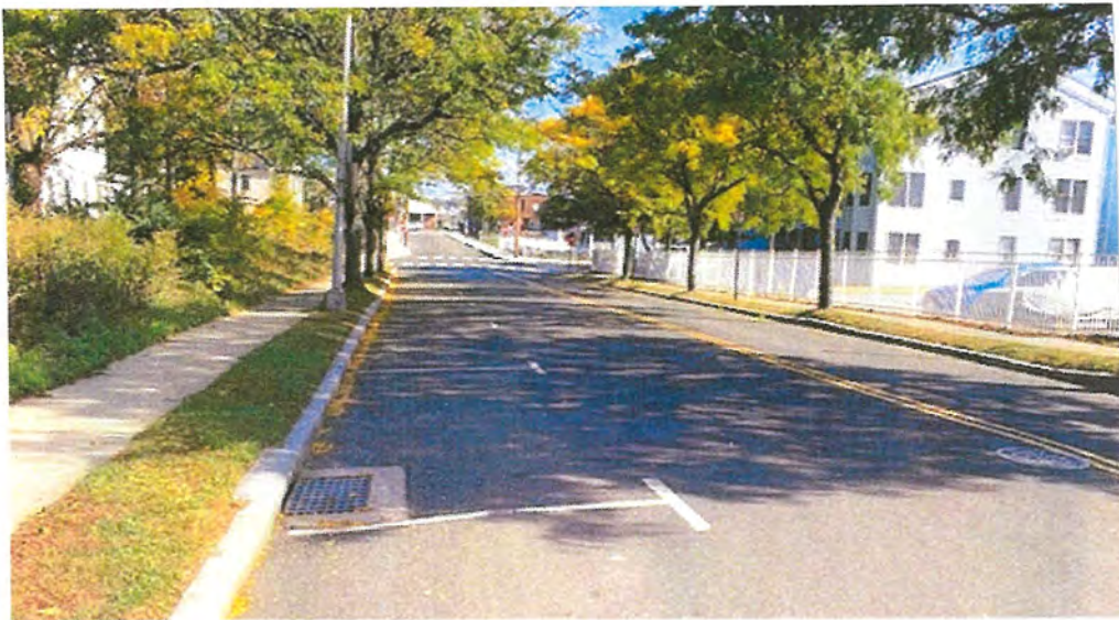
Henry Street Extension Facing East
