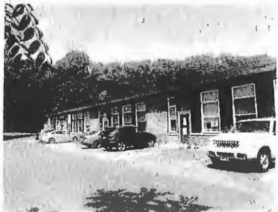
West facing view of existing classrooms
