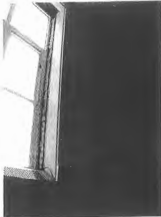
Existing Window Trim Detail
