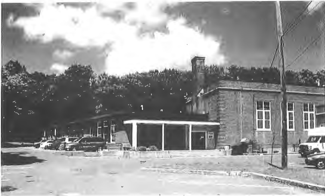
▲ Former Roosevelt School • 11 Allen Road • Norwalk CT
