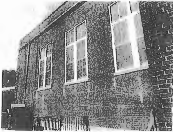
South facing view of existing Gymnasium
