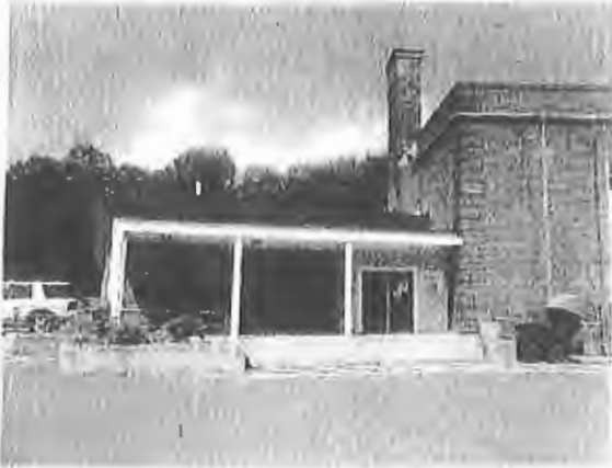
Existing/Proposed Main entry - Looking North
