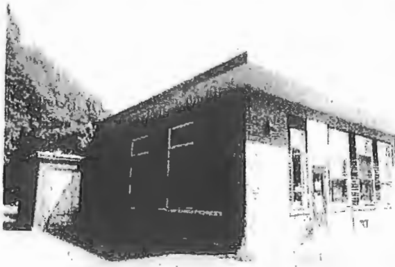
North-West corner of existing classroom
