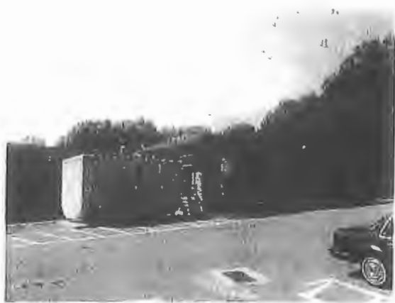
South-East view of existing Classroom
