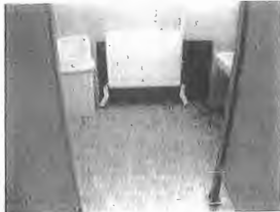
Typical toilet Room
