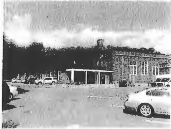
Existing/Proposed Main Entry – Looking East
