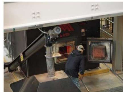
Figure 52. Examples of urban wood waste utilization from left to right: Portable sawmill processing a high-value cherry log; a mulch yard in Southington; a wood chip burning firebox at Hotchkiss School where the wood ash is then used as a soil amendment (Source: CT DEEP Division of Forestry, June 2014)
