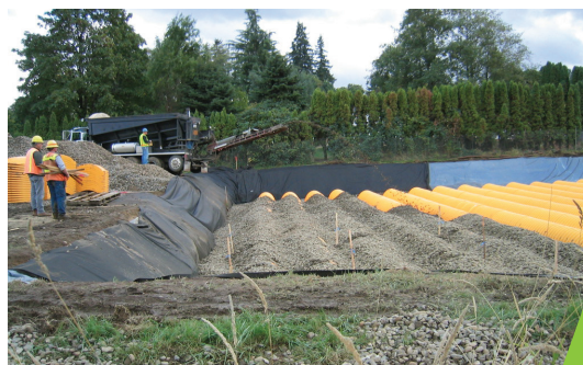
Angular stone backfill is placed around chambers.
