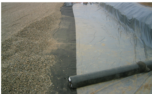
Non-woven fabric is placed over PVC liner before placing angular bedding stone.
