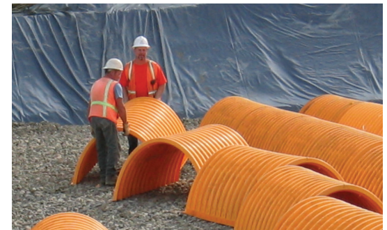
The membrane's flexibility is apparent by visible wrinkling. Flexibility enables the liner to conform to irregularities in the excavation and resist puncture.
