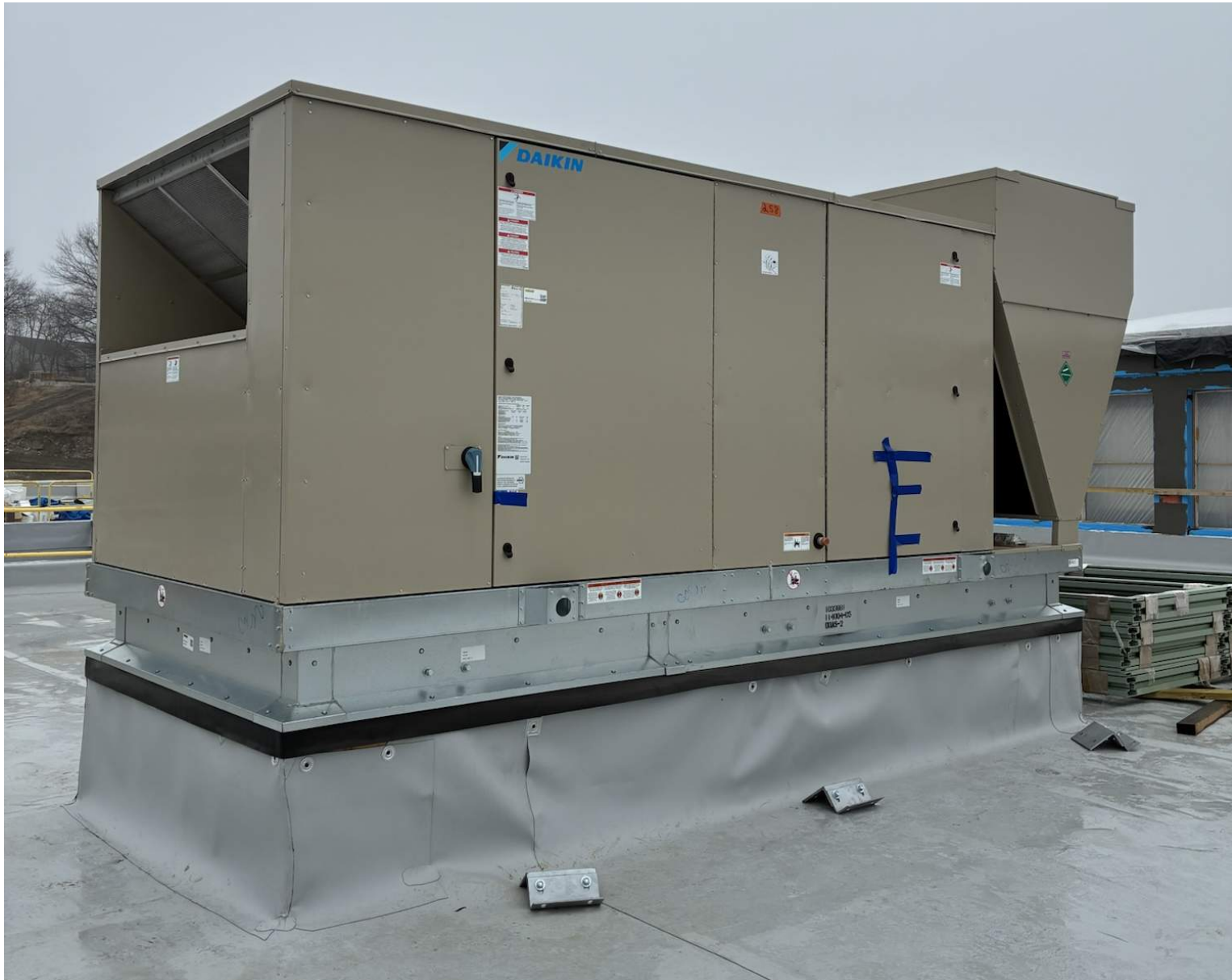
Rooftop Unit Set & Curtainwall Frames for Main Stair 3/20/25
