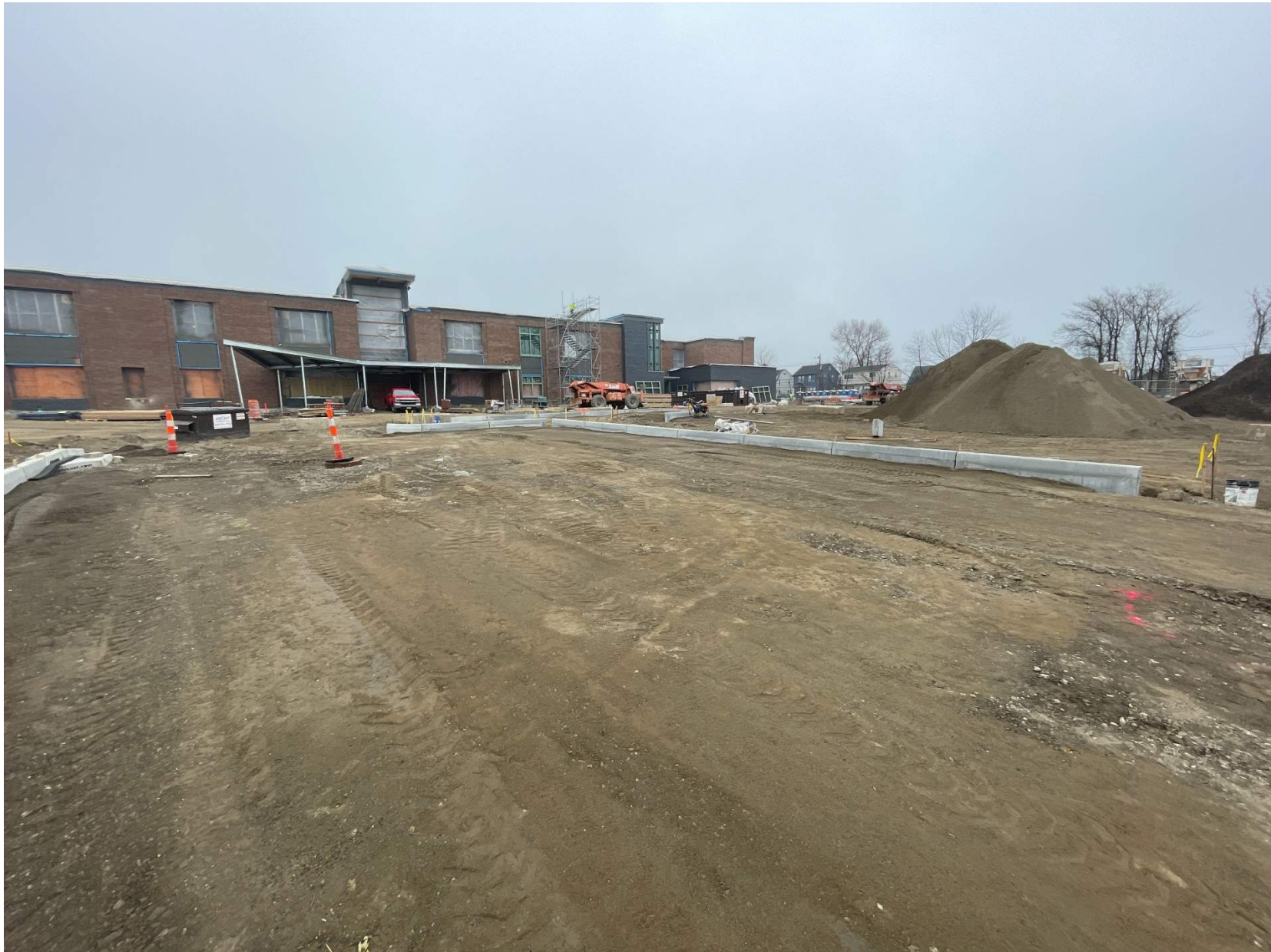
Main Entrance on South Elevation & Parking Lot Grading w/ Curbs 3/15/25
