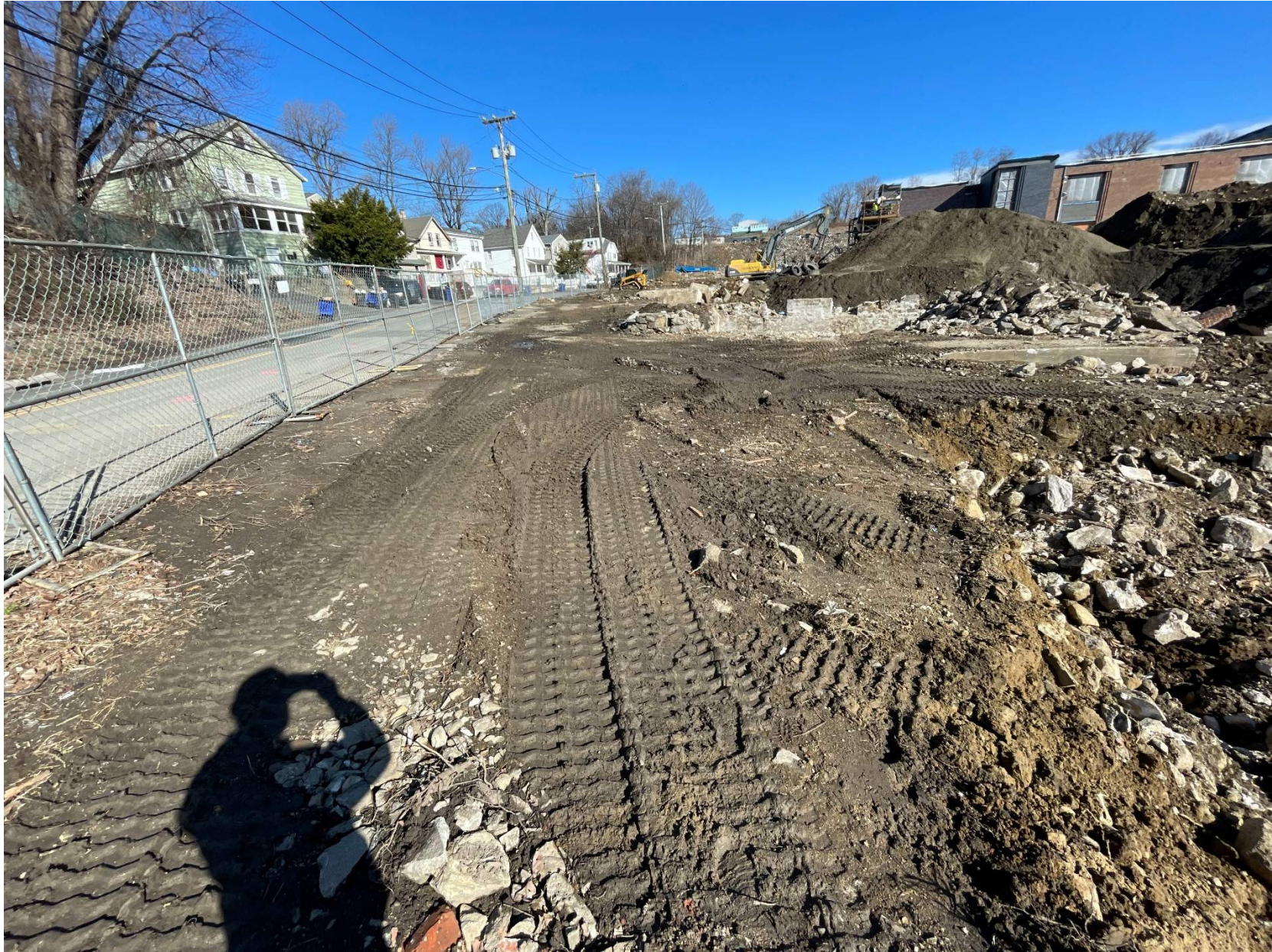
Demolition on Oxford Properties 3/18/25
