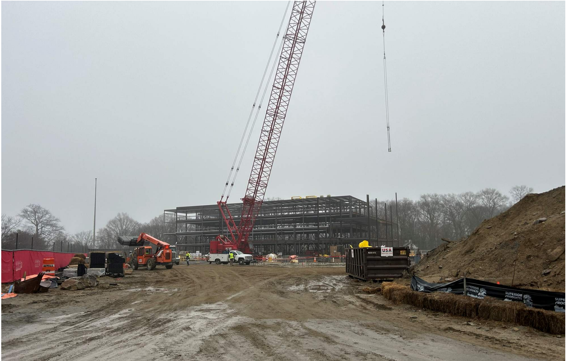
Crane, Steel Erection 3/20/25
