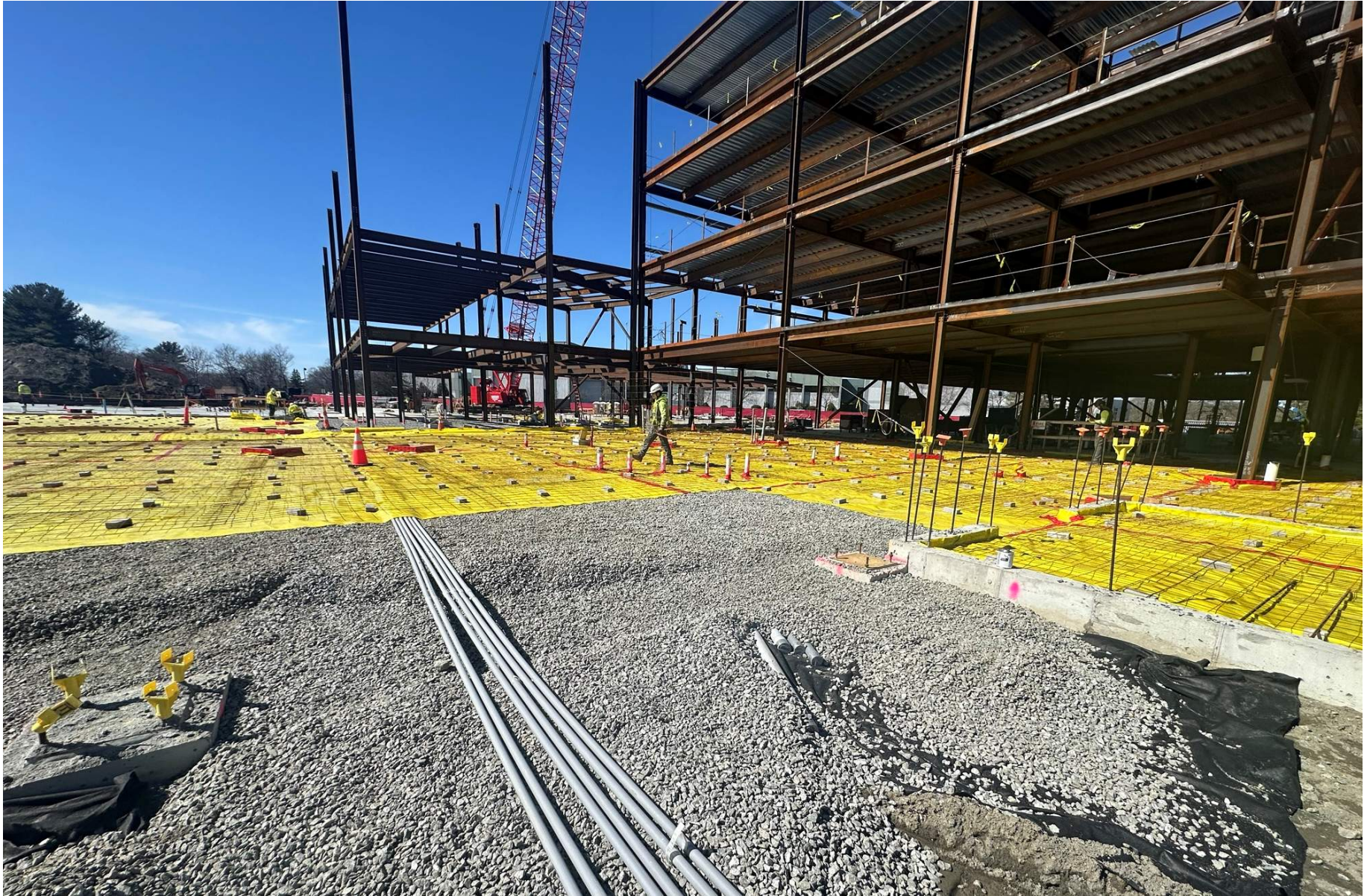
Steel Erection, Slab on Grade Prep, Underground Utilities 3/20/25
