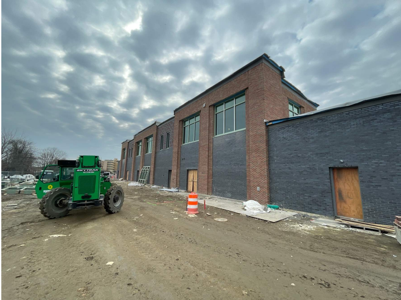
Service Area Elevation on East Side 3/4/25
